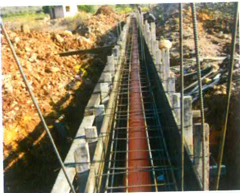
Suspention beam for protection of 10" line –Baqa
