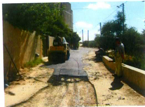
Asfalt work – Baqa
