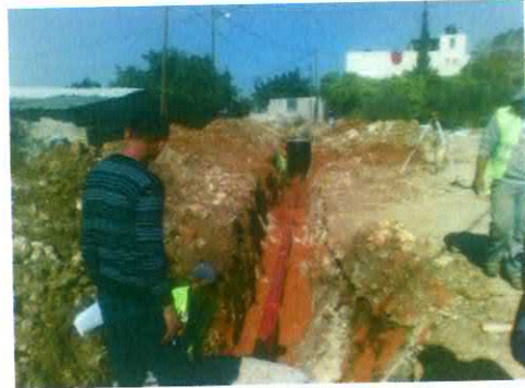
Installation of 8" UPVC pipe lines Barta'a
