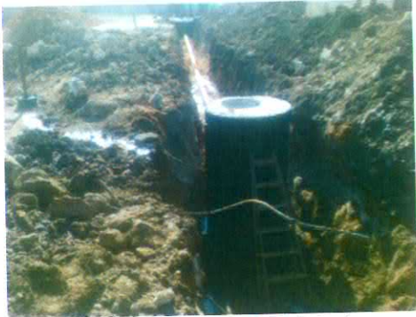
Installation of Manhols –Barta'a
